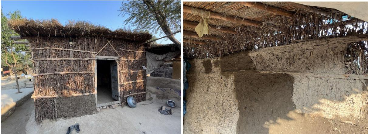
Traditional massive mud building (cob = straw/mud mixture); section of a collapsed cob house
