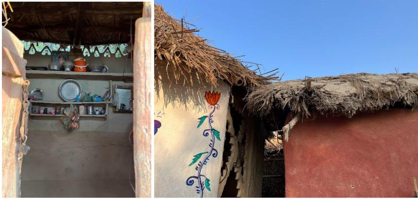
Traditional roofing with wooden beams and a decorated ventilation opening between roof and wall
